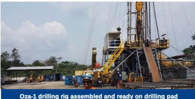
Oza-1 drilling rig assembled and ready on drilling pad
