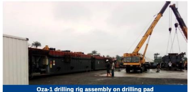
Oza-1 drilling rig assembly on drilling pad
