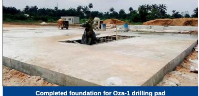
Completed foundation for Oza-1 drilling pad
