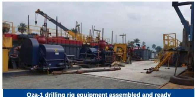
Oza-1 drilling rig equipment assembled and ready
